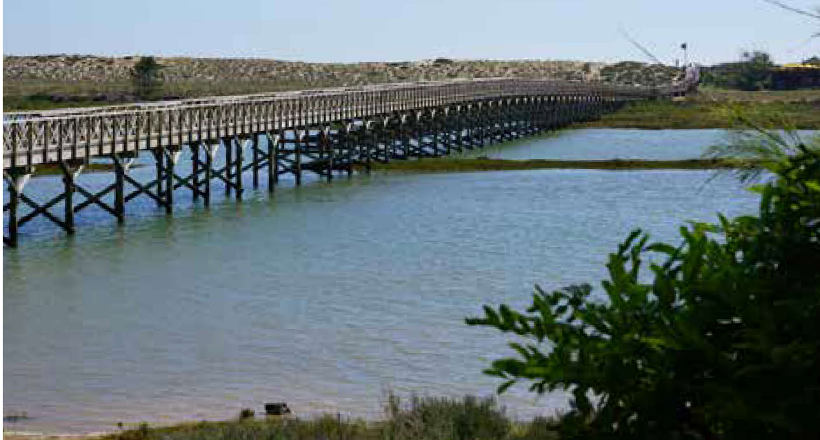
Access bridge to the Ancão beach, at the beginning of the trail
